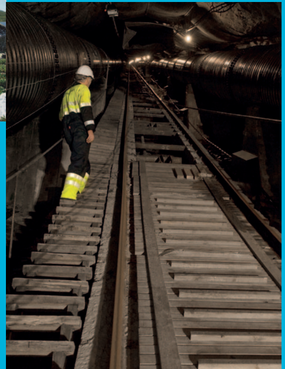
The world's longest wooden stairway, at Mår power station - 3 875 steps
